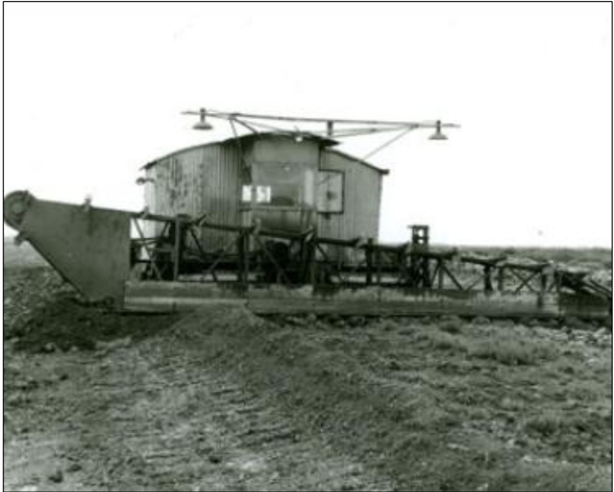
Plate 4-7 Levelling Machine Type - Scraper (Source: Living History)
