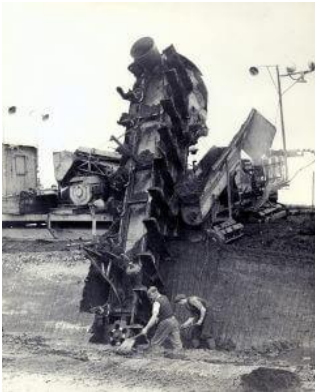
Plate 4-23 Sod Peat Bagger/Excavator (source: Living History)
