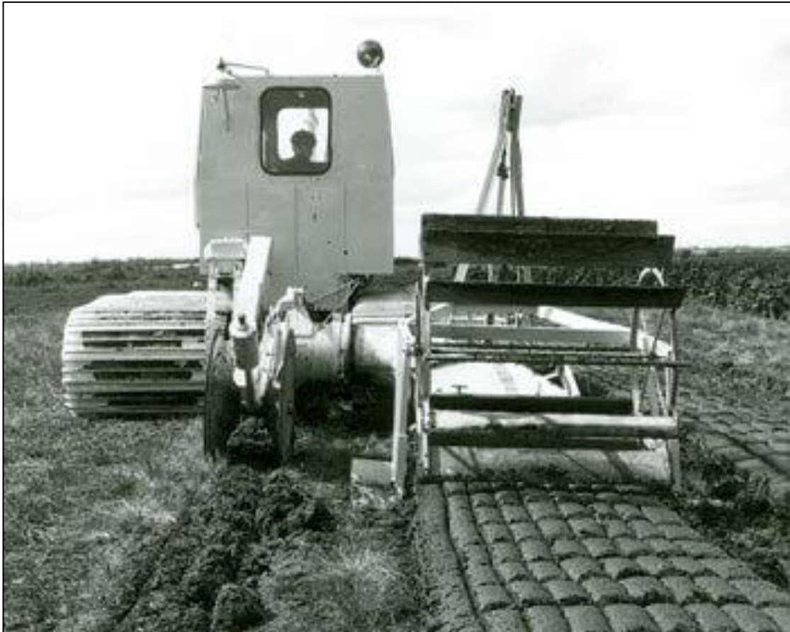
Plate 4-26 Chain Saw Excavator (source: Living History)
