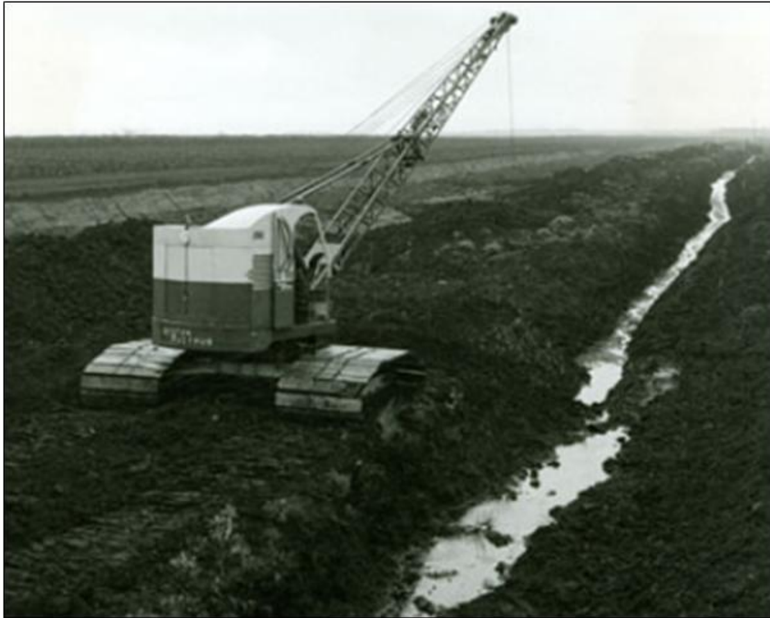
Plate 4-1 Dragline/Shovel excavator (Source: Living History)
