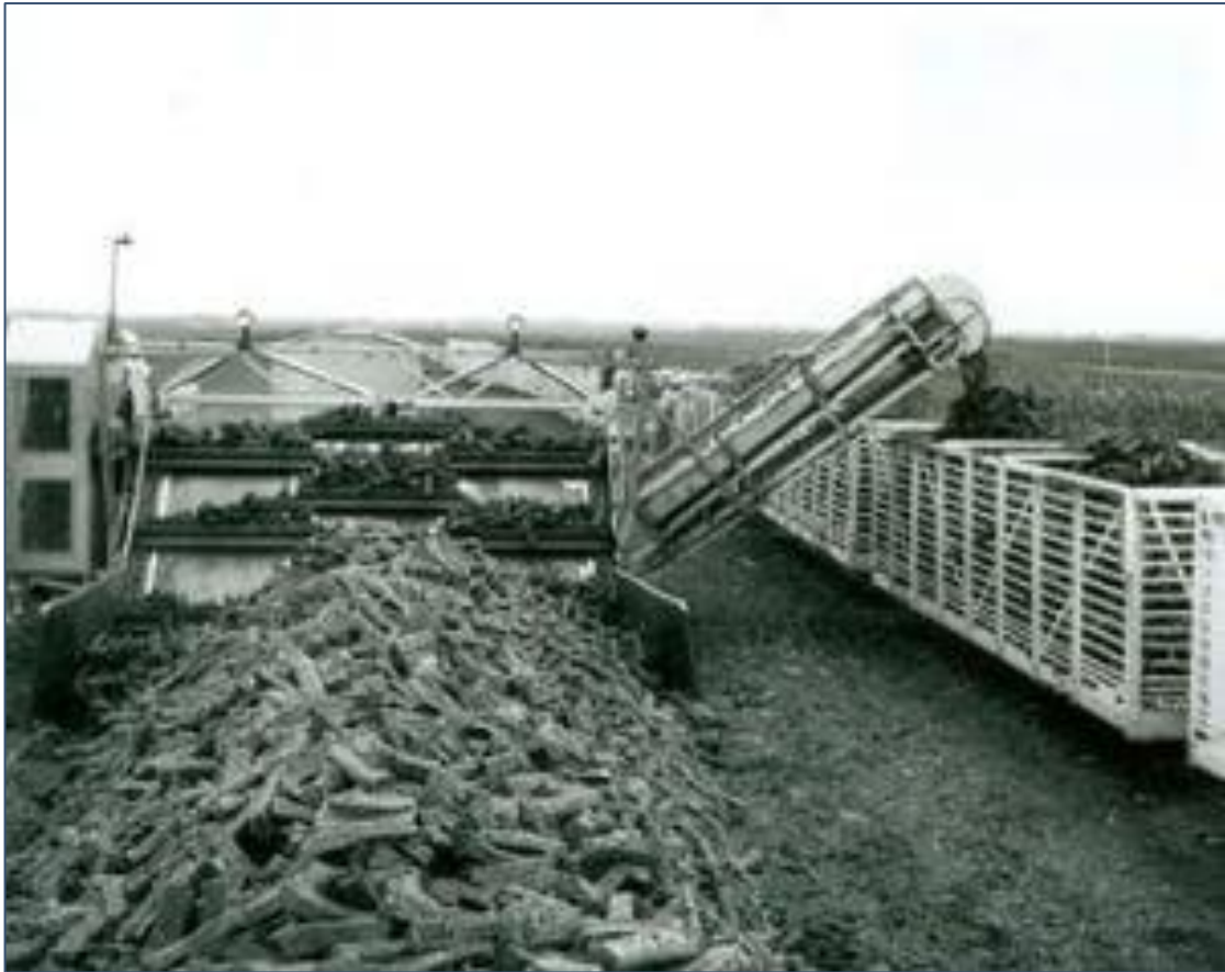
Plate 4-28 Sod Peat Loading Machine (source: Living History)
